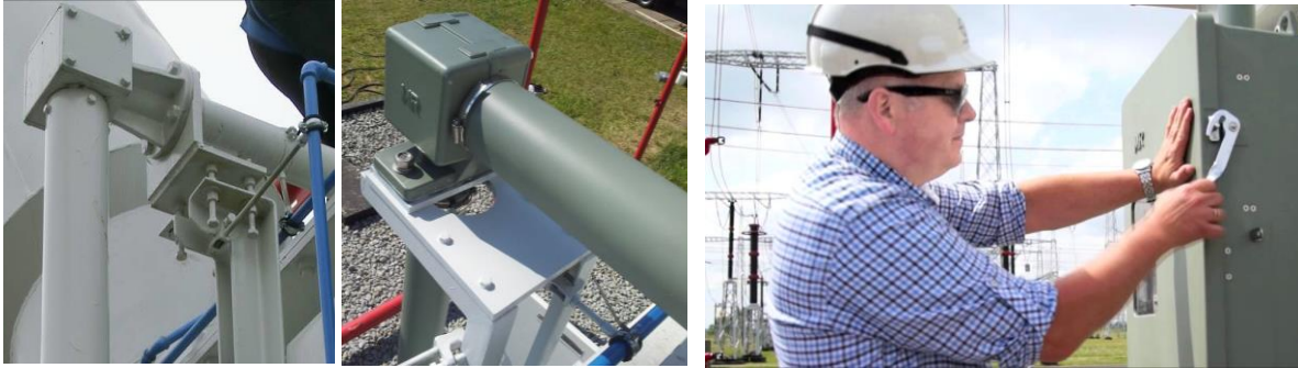
Fig. 4. Original and replaced angle-transmission of OLTC drive. The new OLTC drive.
